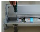
3. Connect the power cable to the right terminal through the cable gland
